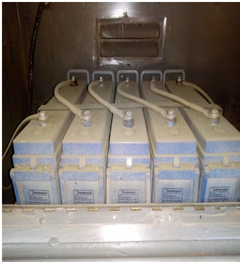
Installed & Maintenance of VRLA, LMLA Battery at Indian Railways (Southern Western Railways)
