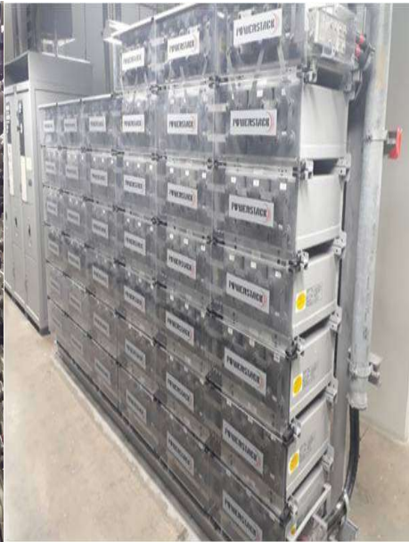
VRLA Battery I&C at BMRCL
