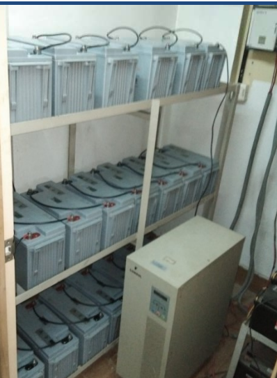
Installed Quanta 150AH Battery at Banks to Branch Office & ATM Location
