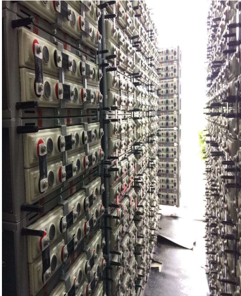
VRLA Battery I&C at Telecom
