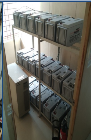
Installed Quanta 150AH Battery at Banks to Branch Office & ATM Location
