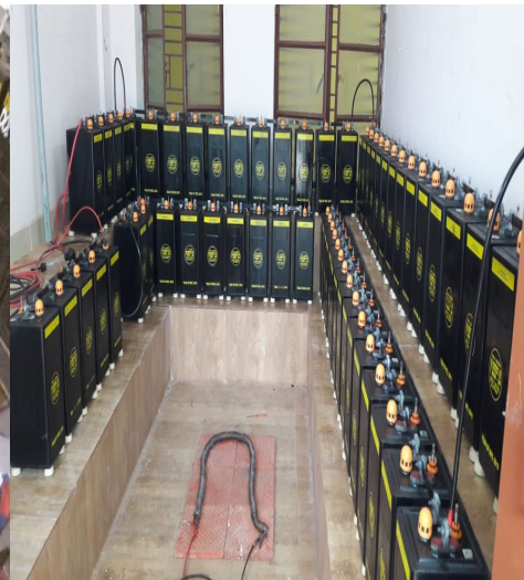
Installed & Maintenance of VRLA, LMLA Battery at Indian Railways (Southern Western Railways)
