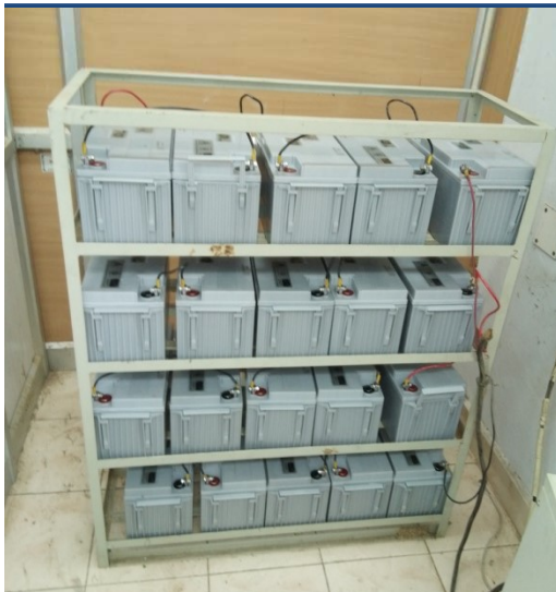
Installed Quanta 150AH Battery at Banks to Branch Office & ATM Location
